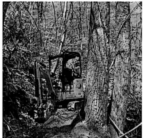
Construction Of Gateway Trails 2024
