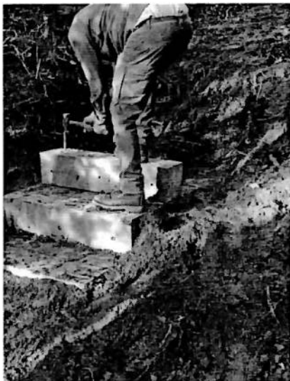
Timber Box Step Construction, Bartram Trail
