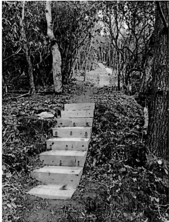
Timber Box Step Construction, Bartram Trail
